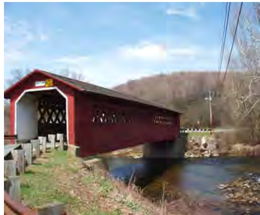
The Henry Covered Bridge is one of three historic bridges spanning the Walloomsac River.
