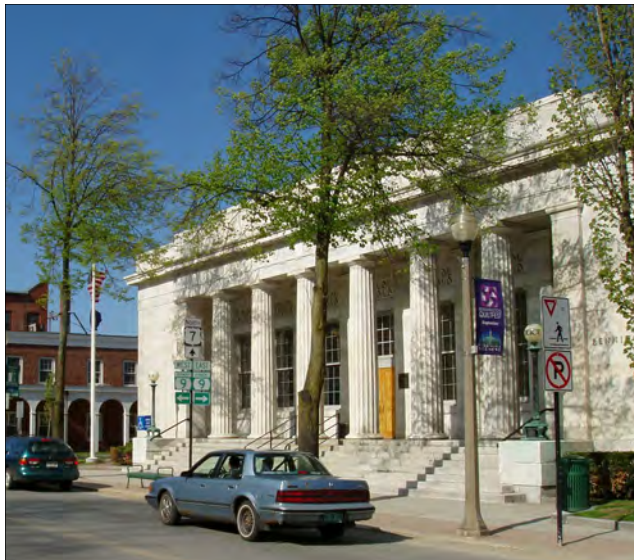
The Police Station must remain active around the clock every day, contributing to a high rate of electricity usage.
