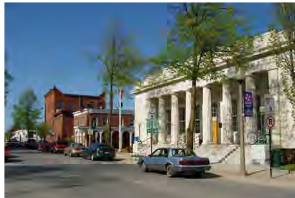
There is a concentration of important historic structures in the Downtown Historic District; the former Federal Building is in the foreground of this photograph looking up South Street.
